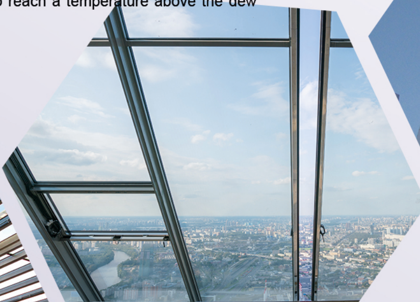
Electrically heatable FGL heated glass on top and sloped areas. Mercury City Tower, Moscow. Customer Josef Gartner GmbH Germany.
